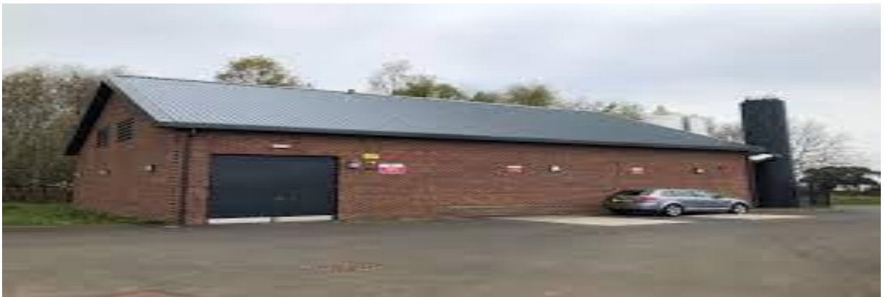
Image of District Heating System Plant Room located to the rear of West Whitlawburn HC Offices
