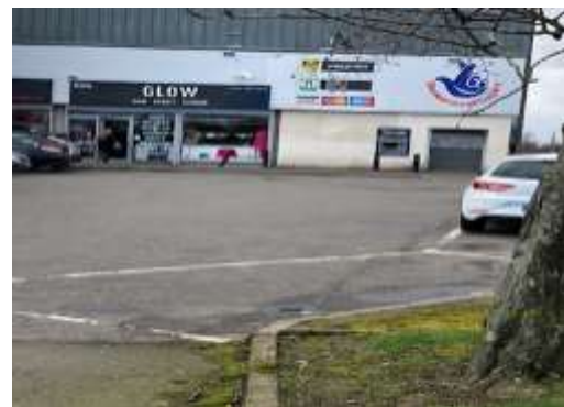
Photograph taken Mid-March
